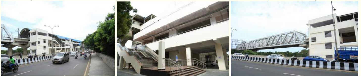
Guindy Metro Station
