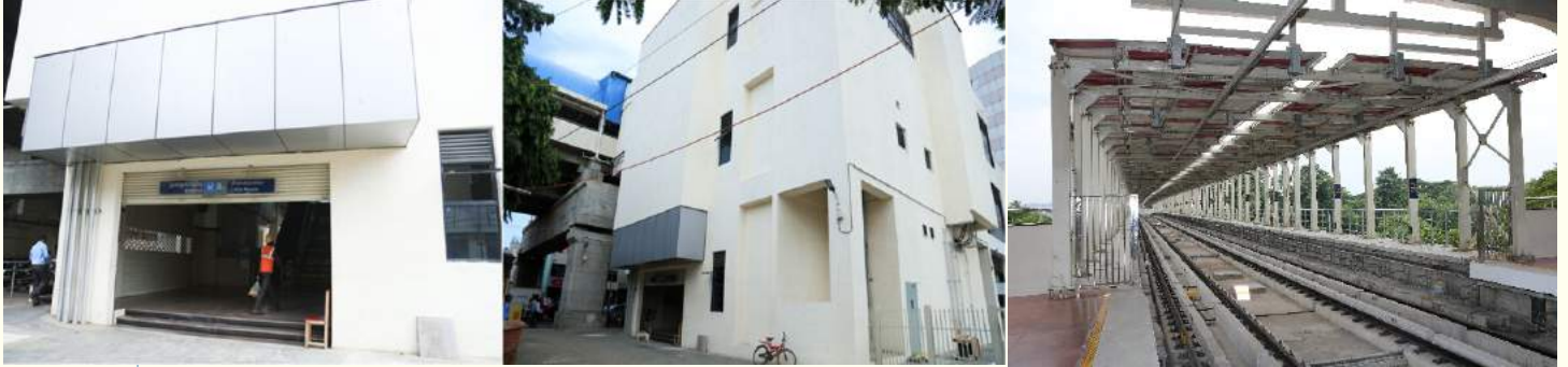
Little Mount Metro Station
