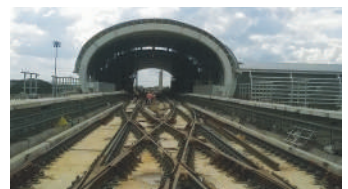
Diamond cross over track work completed at Airport station
