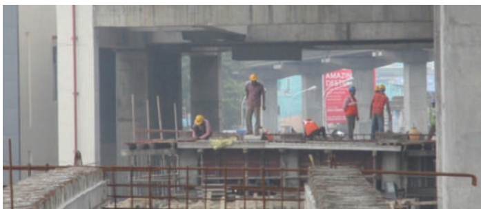
Work in progress at Vadapalani Flyover
