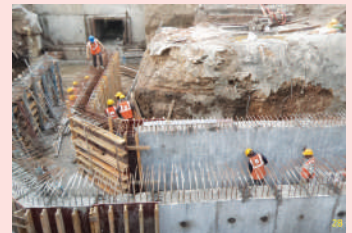
Utility gallery rebar work in progress at Nehru Park Station
