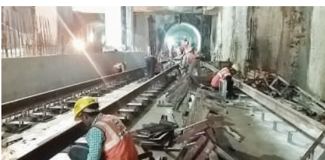
Diamond crossing grouting work in progress at Shenoy Nagar Metro Station
