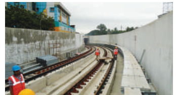
Track work completed at Thirumangalam ramp
