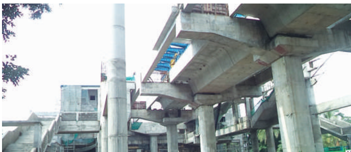
Work in progress at Meenambakkam towards Airport Viaduct
