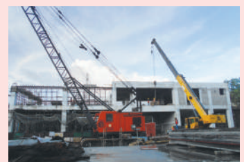
Work in progress at Anna Nagar East Station
