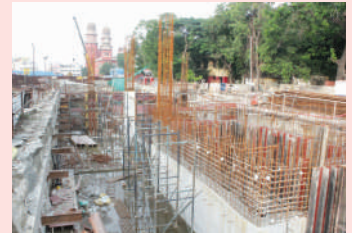
Work in progress at High Court Station
