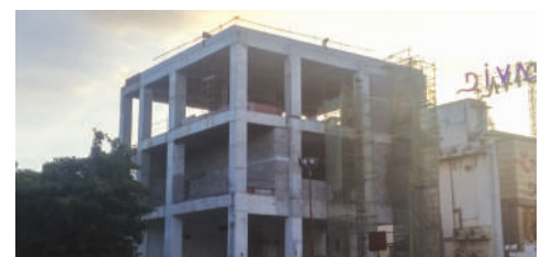
Work in progress at Anna Nagar Tower Station
