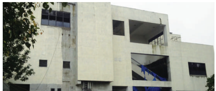
Work in progress at Little Mount Station
