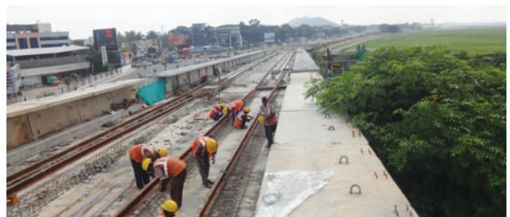
Work in progress from Nanganallur Road to Airport
