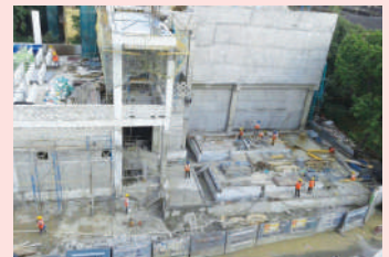
Ancillary building DG area work in progress at Pachaiyappa's Station
