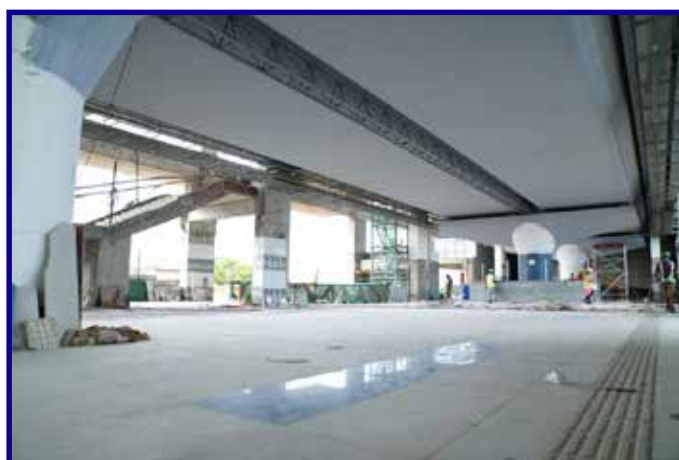
Concourse level finishing works in progress at Wimco Nagar Metro Station
