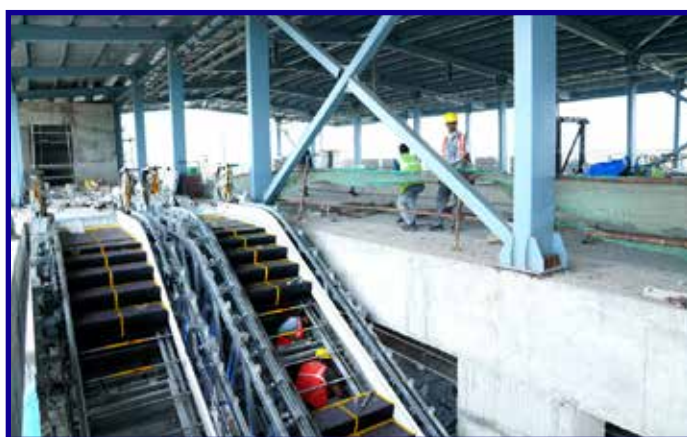
Escalator fixing work at Wimco Nagar Metro Station
