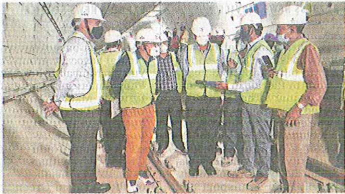
Commissioner of Metro Railways Safety Abhai Kumar Rai inspecting the phase-1 metro rail extension stretch from Old Washermenpet to Wimco Nagar on Friday
