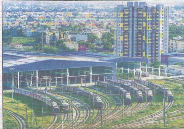
POINT OF RETURN: The existing metro rail depot at Koyambedu
