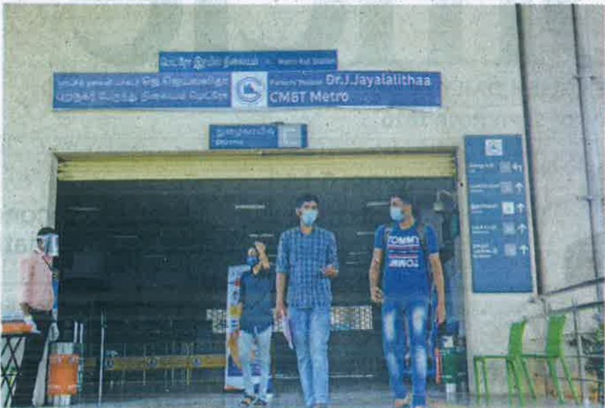
The CMBT metro rail station renamed as 'Puratchi Thalaivi Dr J. Jayalalithaa CMBT metro.' - DC
