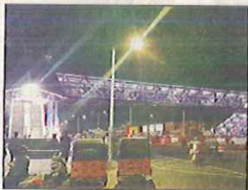
The foot over-bridge has escalators and elevators
