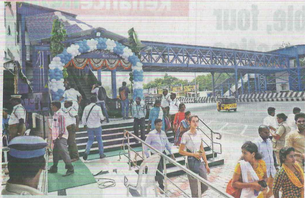
The FOB has CCTV cameras and LED lights to ensure safety along with a ramp to help the physically challenged people to make use of the lift facility
