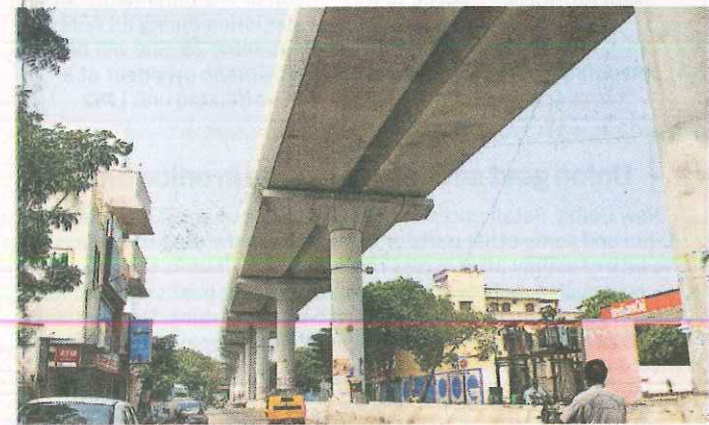
Metro Rail work in progress at Tiruvottriyur High Road | D SAMPATHKUMAR
