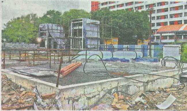
The subway construction under way on EVR Periyar Salai
