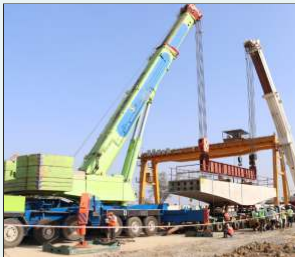
Stacked U Girder & lifting of Pier cap at Casting yard
