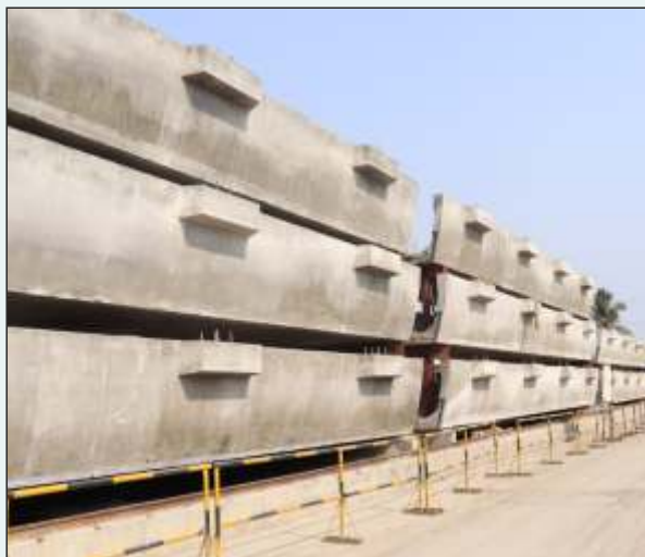
Stacked U Girder & lifting of Pier cap at Casting yard
