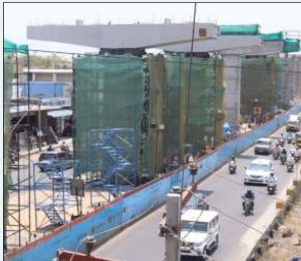
U Girder Erected at Porur site
