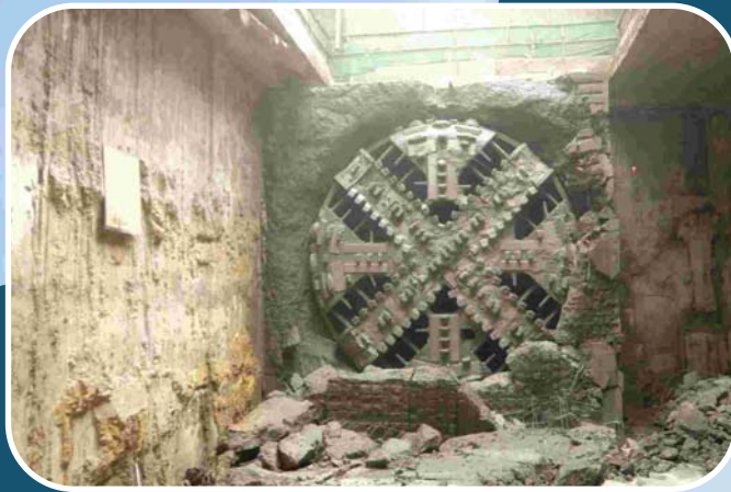
D-Wall break through at Kilpauk
