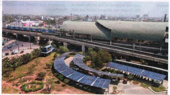
Chennai Metro Rail Ltd (CMRL) has made good use of its vehicle parking spaces and station rooftops to install solar power panels and generate around 1.51 lakh units every month. It is expected to save around ₹70 lakh in power bills annually. Panels have been installed on the roofs of two elevated stations — Alandur and St Thomas Mount Metro — and on the ground level at Metro Rail Depot, Koyambedu. By the year end, around 8 MW of solar power capacity will be installed, says CMRL BIJOY GHOSH
