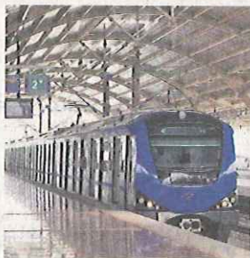
The Phase I extension of Metro is estimated to cost ₹3,770 crore.
