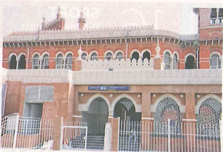
High Court metro railway station nearing completion.
