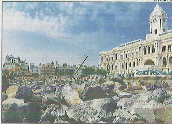
WORK IN PROGRESS: The stretch near Ripon building will be relaid
