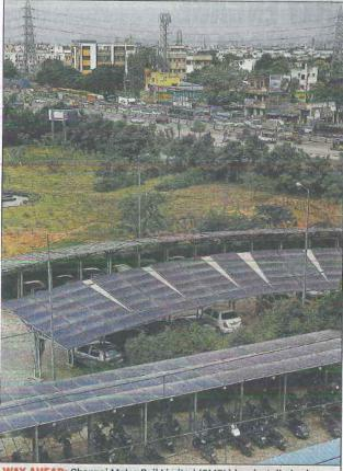
WAY AHEAD: Chennal Metro Rail Limited (CMRL) has installed solar panels on the roof of the parking lot in its Koyambedu headquarters. The CMRL has more than 1MW capacity solar panels in its head office and maintenance depot. Power generated from these panels is used for train maintenance and lighting purposes. It also has solar panels in its various stations with a total installed capacity of 2.1MW
