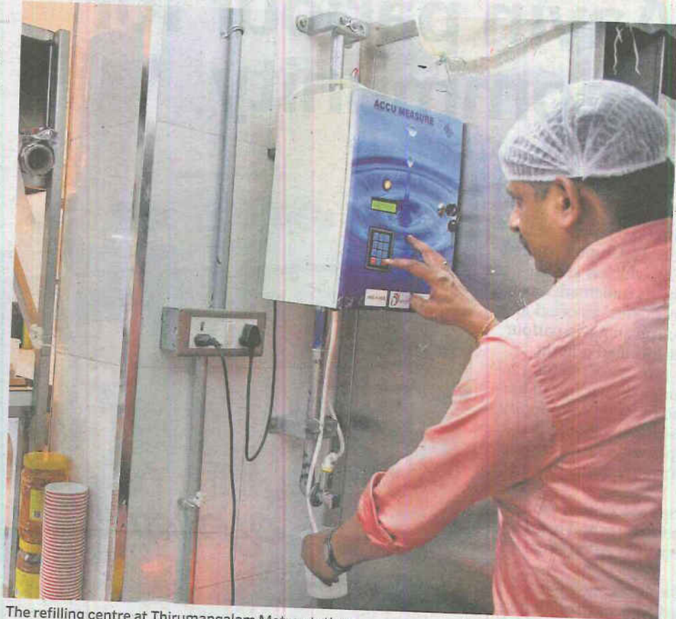
The refilling centre at Thirumangalam Metro station.
