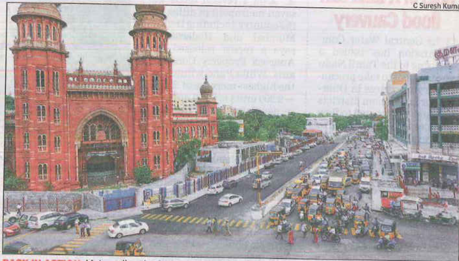
BACK IN ACTION: Metro rail authorities handed over the road to the traffic police last week
