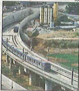
In automatic train protection mode, the metro services are operated manually
