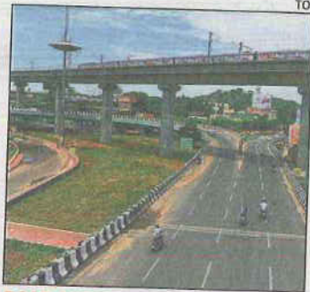
ROAD AHEAD: Many facilities expected to come up in the 54,400sqm space under the Kathipara interchange
