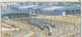
QUICK RESPONSE: At the depot, the software will download the logs daily before a train chugs in for servicing. CMRL has about four hours to service trains
