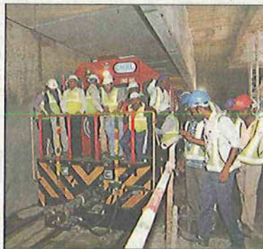
Officials during the 4-km trial run at Little Mount metro station on Thursday
