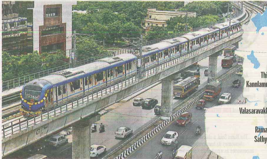
CMRL is set to acquire 86 acres of land for the 55-km stretch for Corridors 3 and 5
