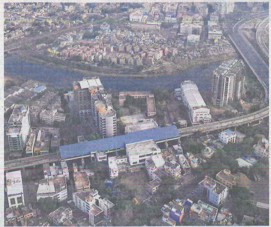
An aerial view of the Saidapet Metro Rail station. ■ B. JOTHI RAMALINGAM
