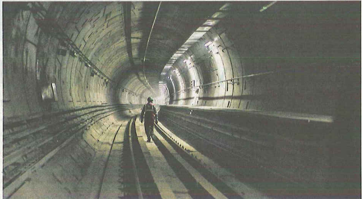
Central link: An employee of the Chennai Metro Rail Limited walks in one of the tunnels between Nehru Park and Egmore in Chennai. This line between Nehru Park and Chennai Central is to be opened by March 2018. •DINESH KRISHNAN
