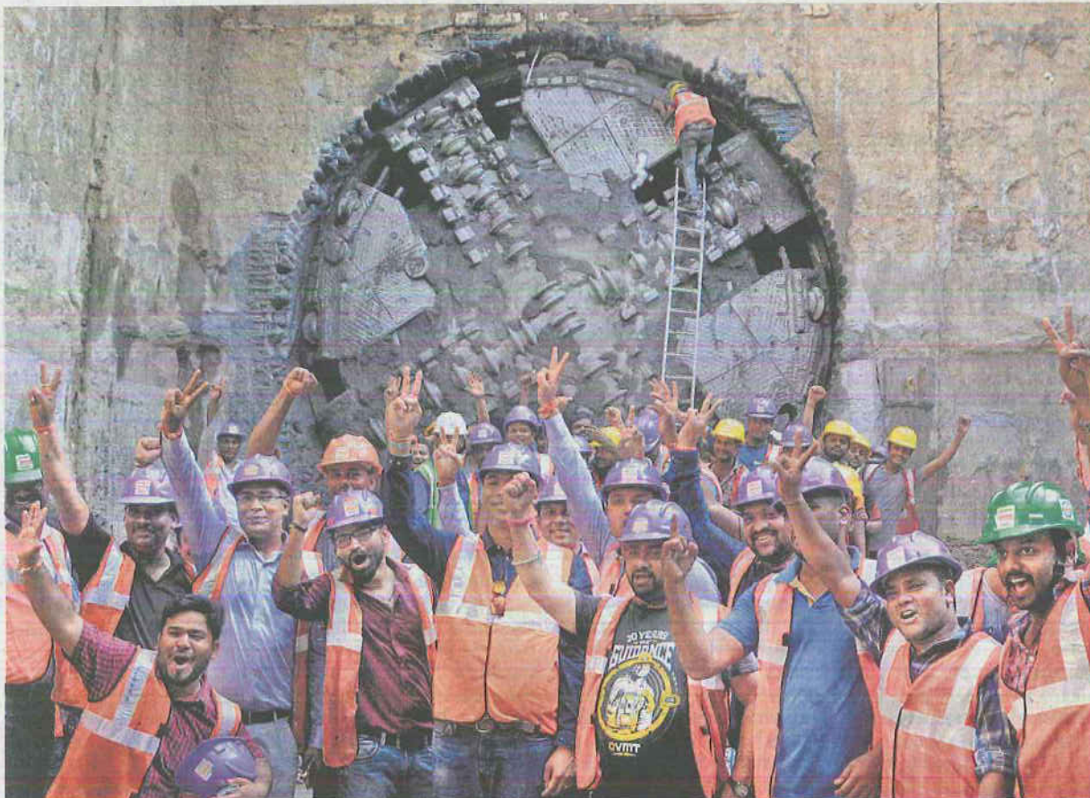
Fruits of labour: Workers celebrate after completing a tunnel as part of the Metro's Phase I extension. ■ B. JOTHI RAMALINGAM
