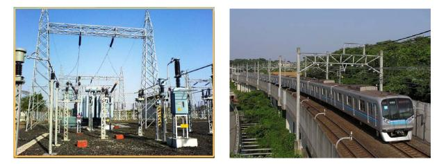
This contract also provides setting up of three auxiliary sub-stations at Koyambedu, Alandur and Chennai Central to step down the 110 kV to 33 kV for supply of power to stations, air-conditioning systems, tunnel ventilation systems, lighting and other utilities at the stations. The sub-stations will be of gas insulated ones for higher reliability and maintenance friendly.
