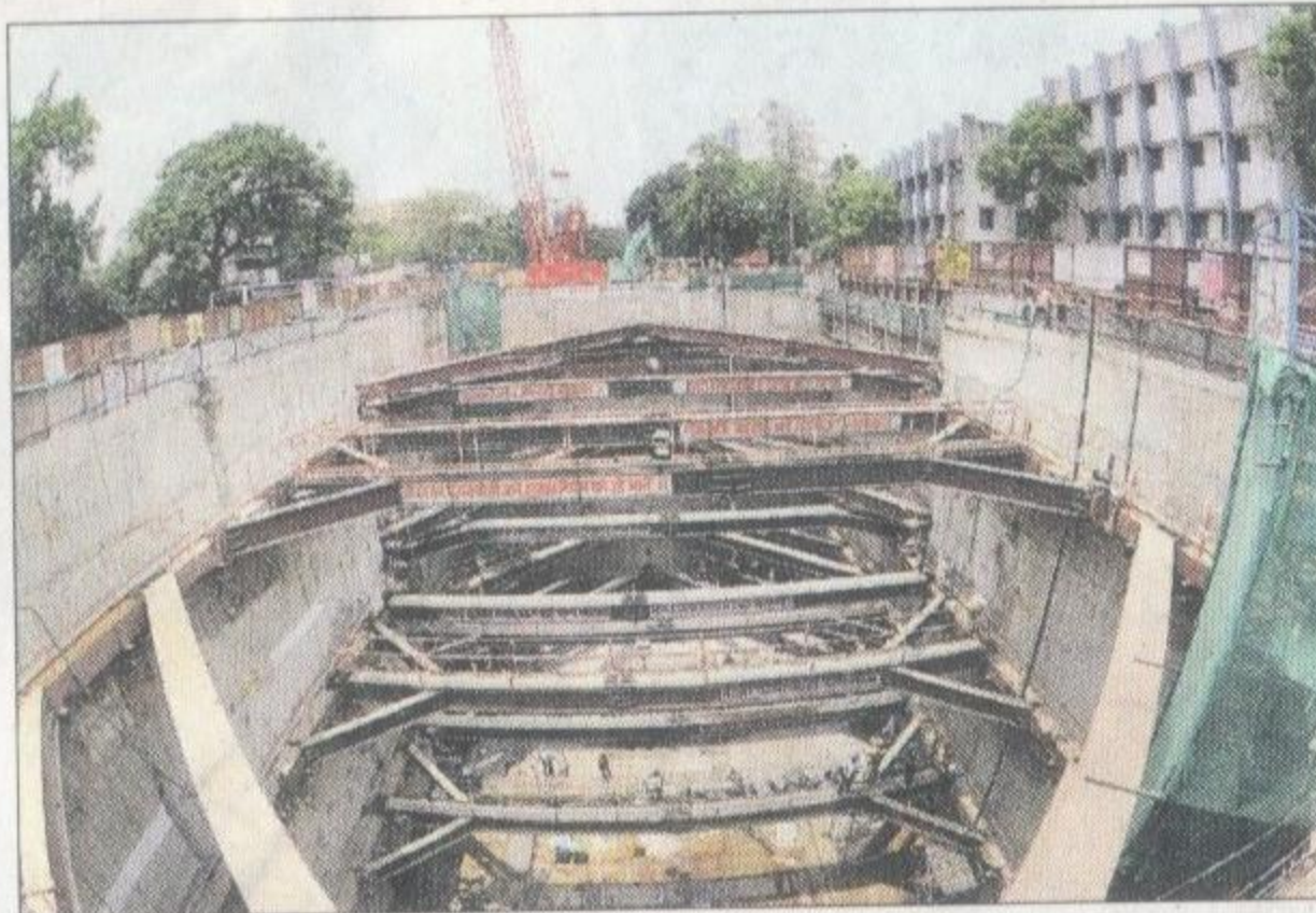
IN PROGRESS: At the site where Nehru Park station will be built, work on the shaft is under way
