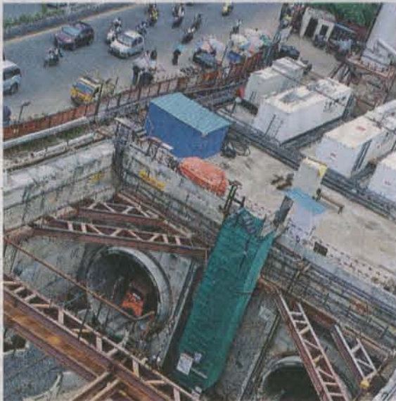
An aerial view of the underground station work at Saidapet.
