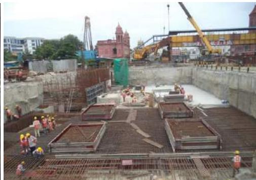
Shaft wall shuttering work in progress
