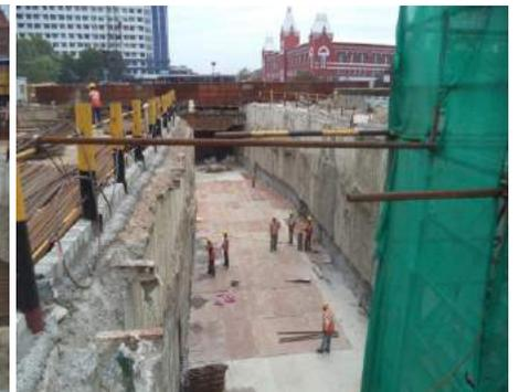
Entry/Exit 02 Roof slab - Rebar Work in progress
