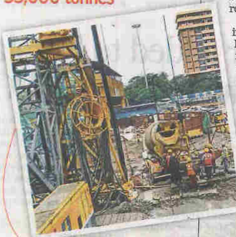
GROUND WORK: Activity during the initial stages at Central Metro
