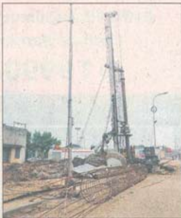
PROMPT START: Ongoing metro work at Koyambedu
