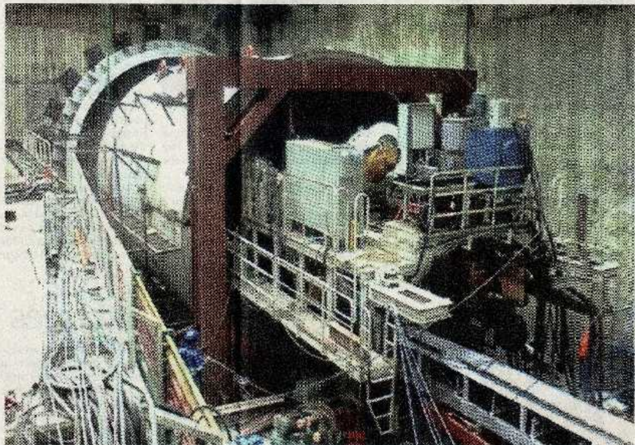
A TBM being lowered into a tunnel on Poenamallee High Road
