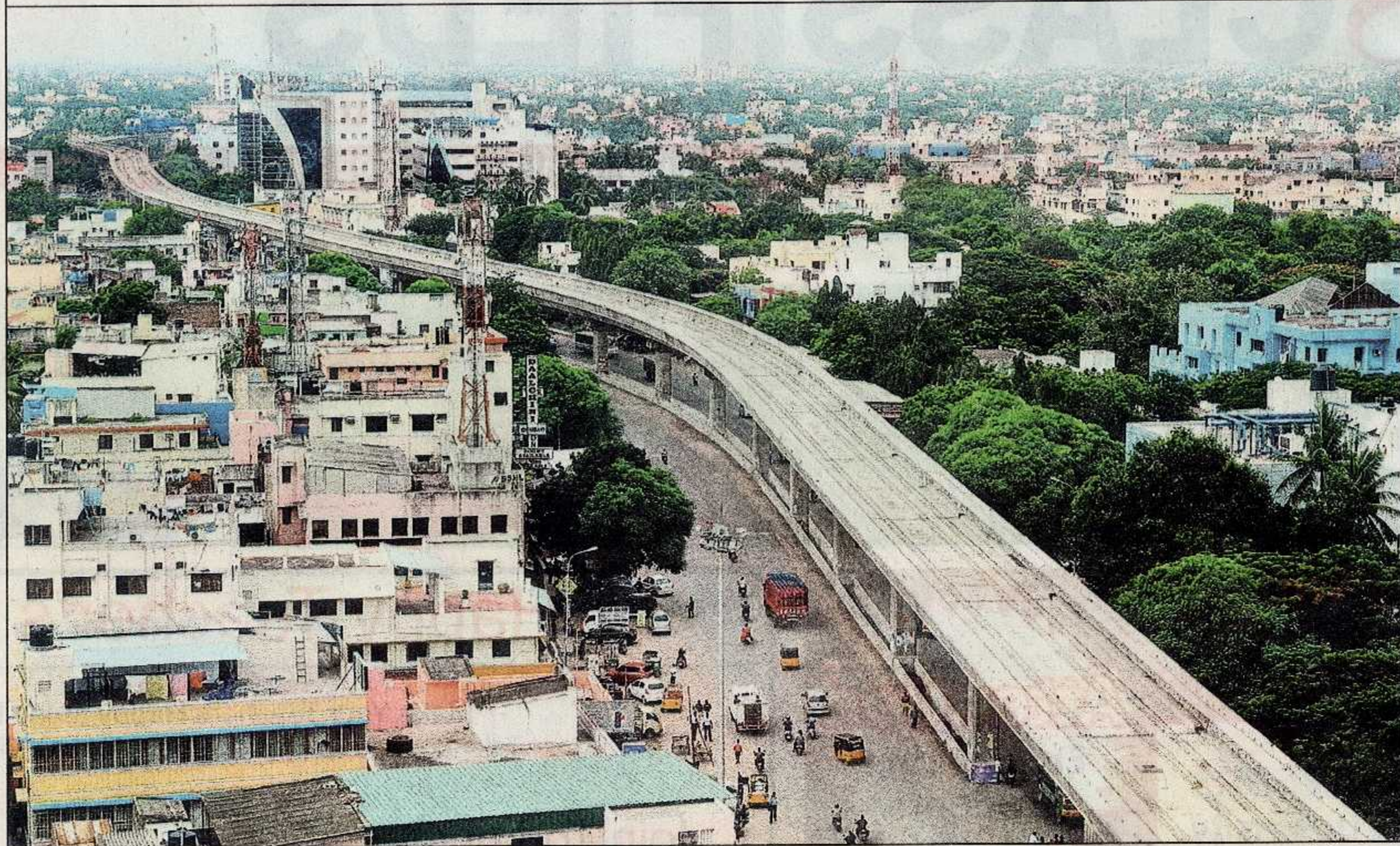
CHANGING CITYSCAPE: Metro rail's elevated corridor snakes over the bustling 100 Feet Road at Ekkattuthangal. The stretch is part of the Koyambedu-St Thomas Mount corridor which is likely to be ready by the end of next year
