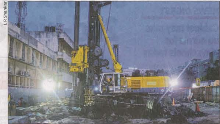
MEANS TO AN END: The grab machine, which excavates soil in order to build the diaphragm wall, in action at the Nandanam signal
