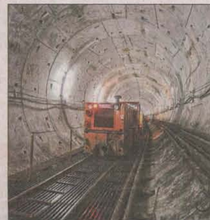
TUNNELS OF TRANSIT: (clockwise from top) The underground tunnel that connects Shenoy Nagar and Anna Nagar Tower stations; the entrance of the tunnel at Shenoy Nagar; the mini-train that helps transport metro rail workers and excavated earth; the tunnel-boring machine at the under-construction Anna Nagar Tower station; a metro rail worker explains the functioning of the control room of a tunnel-boring machine
