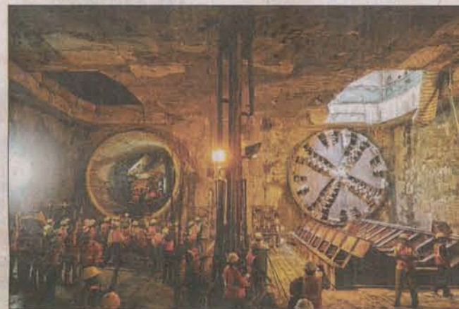
TUNNELS OF TRANSIT: (clockwise from top) The underground tunnel that connects Shenoy Nagar and Anna Nagar Tower stations; the entrance of the tunnel at Shenoy Nagar; the mini-train that helps transport metro rail workers and excavated earth; the tunnel-boring machine at the under-construction Anna Nagar Tower station; a metro rail worker explains the functioning of the control room of a tunnel-boring machine
