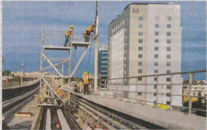
Work on overhead equipment in progress between Little Mount and Alandur
